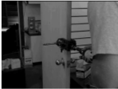
Install new locks
